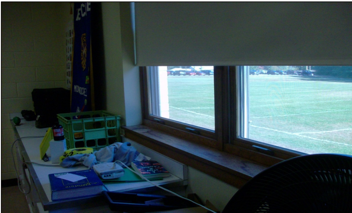
Wood framed, double-hung windows are nearing the end of their useful life.
