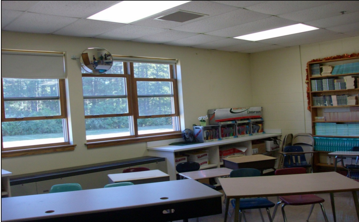
Ceilings, windows, and unit ventilators all need replacement.
