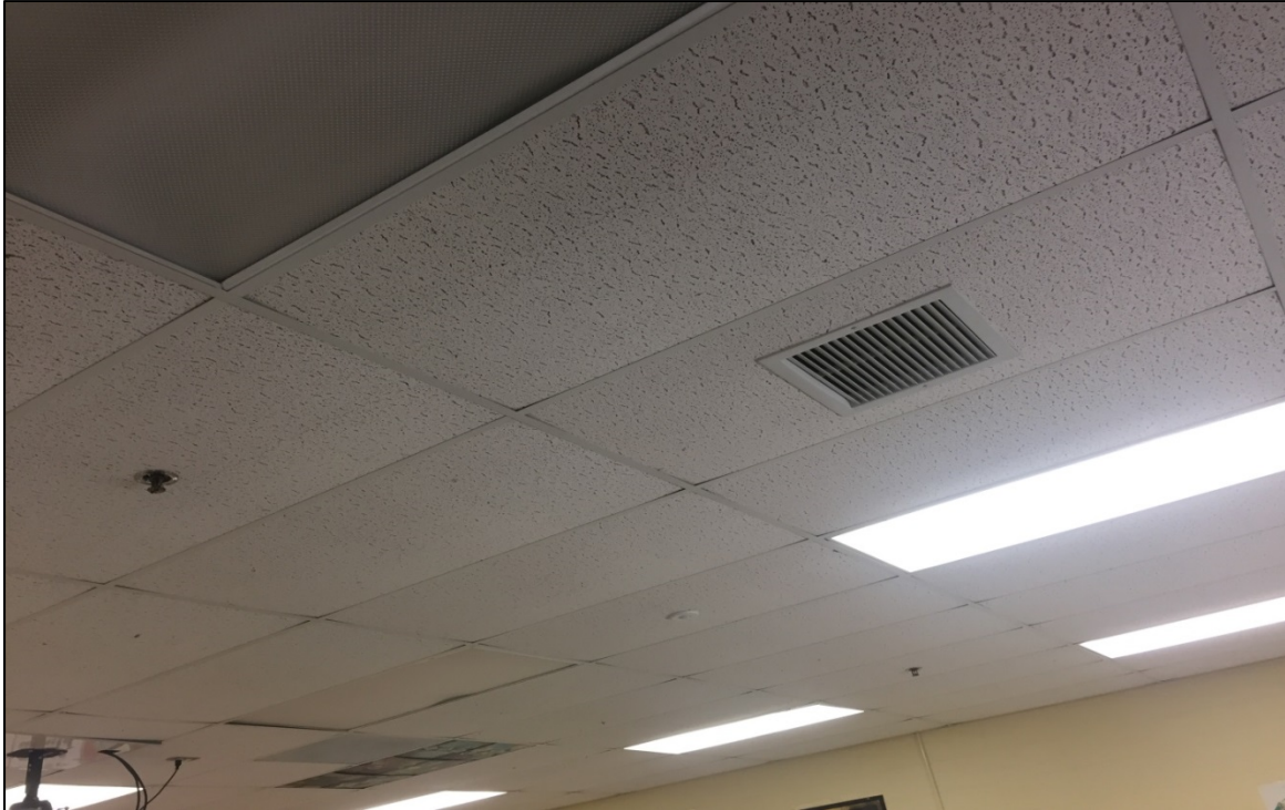
Suspended ceilings are cupped and stained.
