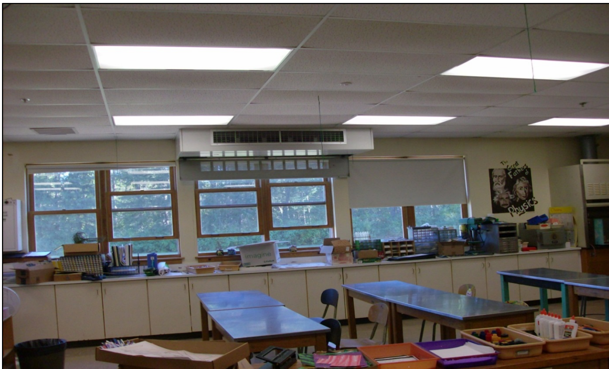
Ceiling mounted unit should be replaced.
